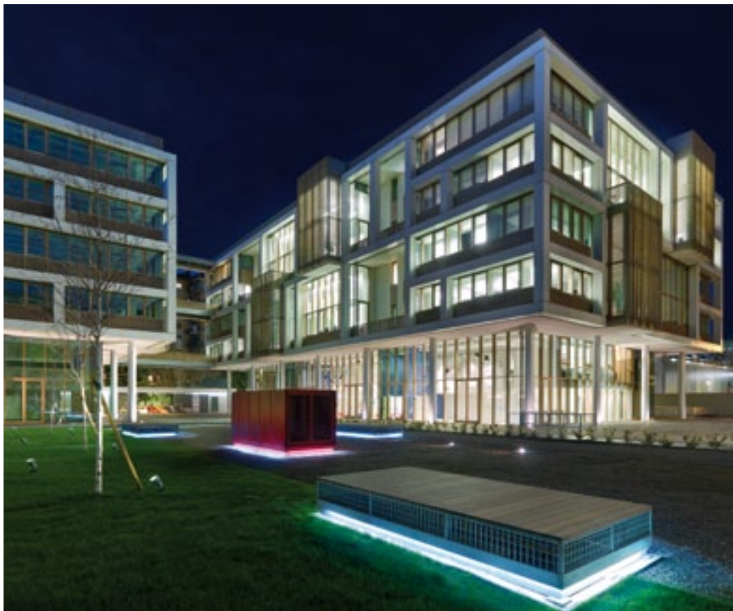
"Tortona 37", Milan, Italy - Arch. Matteo Thun © Entis Illuminazione
